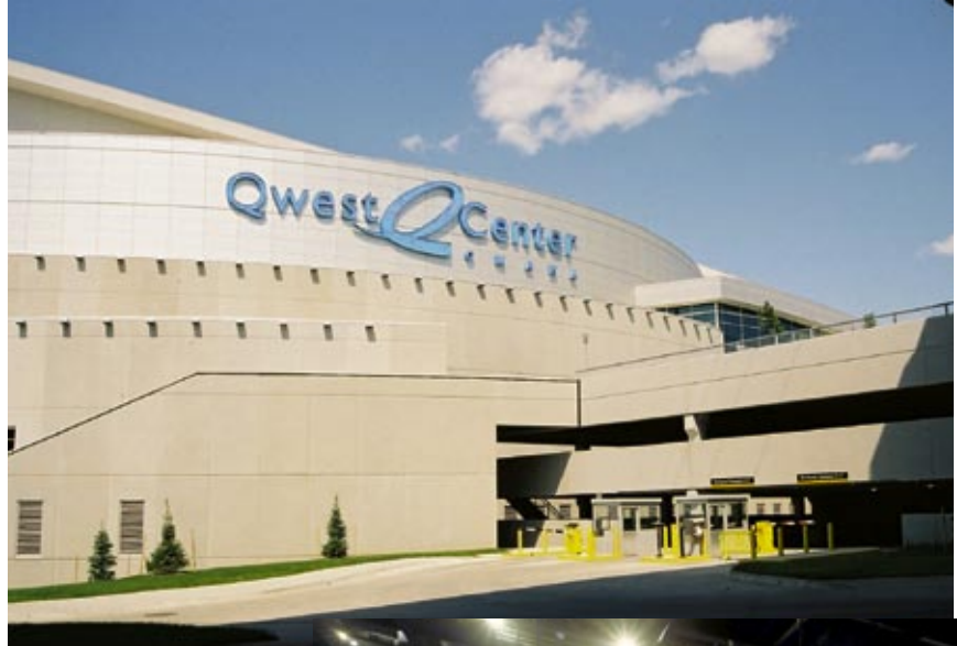
Construction on Quest Center Omaha, which includes both an arena and exhibition hall, took about 2½ years. Precast concrete was used for the exterior insulated panels, vomitory walls and seating decks.
