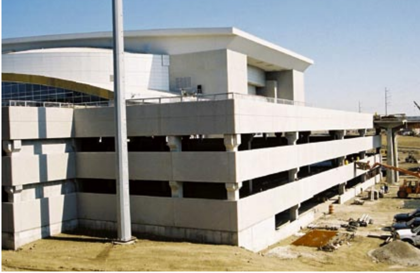
A total-precast concrete parking structure was erected adjacent to the convention center to hold 500 cars. The roof features a grassy, landscaped garden.
